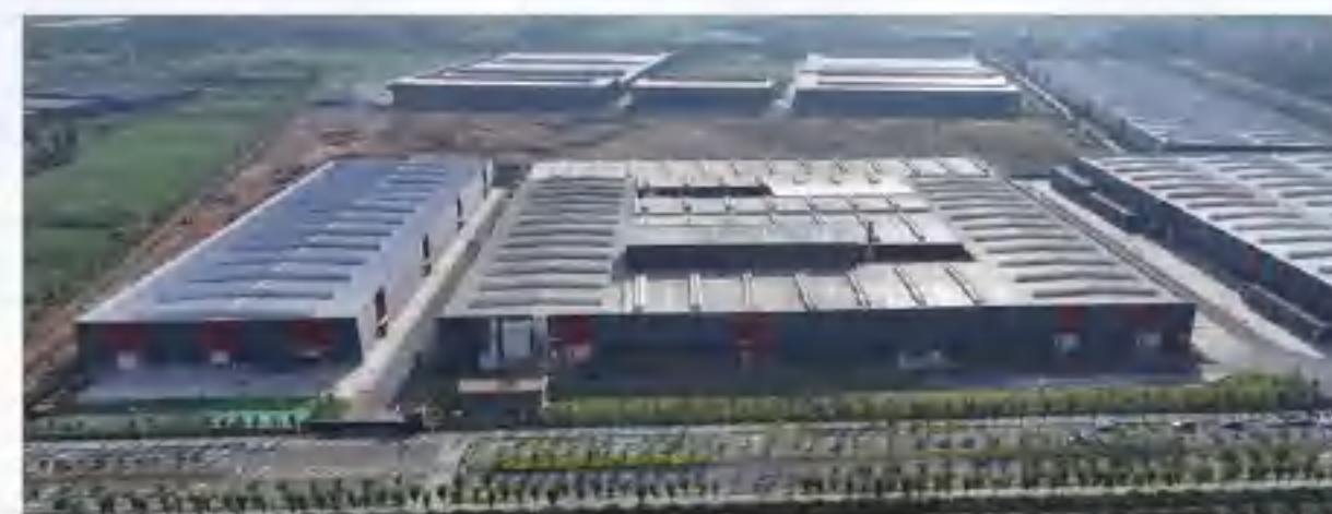
Laohekou, Xiangyang, Hubei, China JK Hubei Re-manufacturing Production Base
